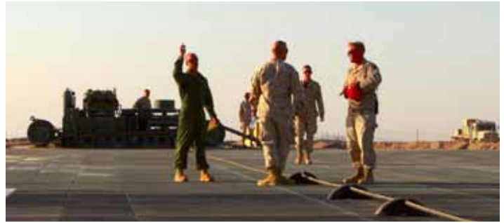
Marines from Marine Wing Support Squadron 274 and Marine Fighter Attack Squadron 232 ensure that the deck pendant, the wire stretched across the landing strip to catch aircraft, is taunt and raised off of the ground before an F/A-18 Hornet uses the newly-installed arresting gear here, June 30.
