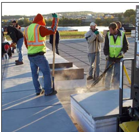
St. Paul Downtown Installation
